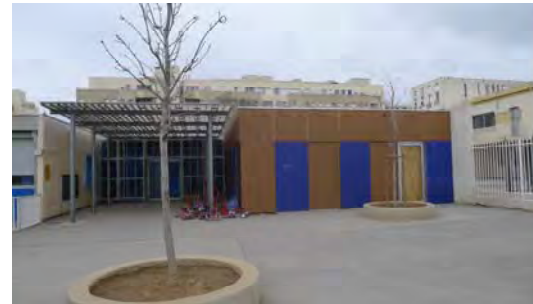
East facades of pre-school (new building)
