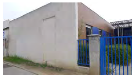
Facade west (cinderblock walls)
