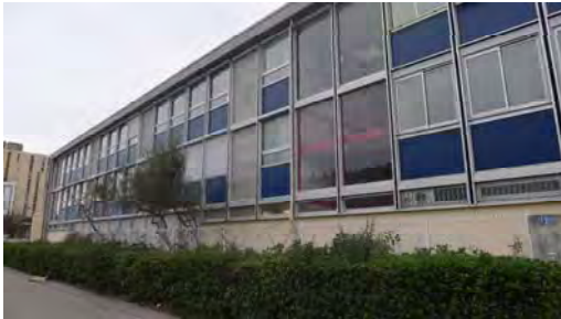
East facades of primary school
