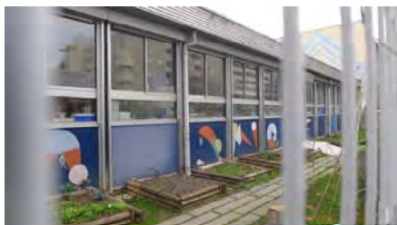
Facade west (panel walls)
