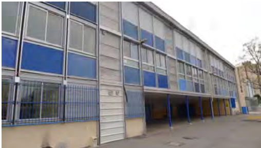
West facades of primary school
